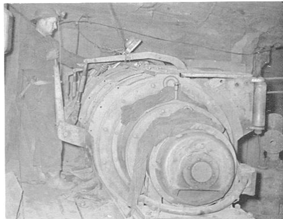
STATIONARY SLUSHER HOIST BEING OPERATED BY BOB LOCKE.
