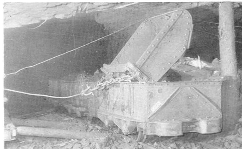
LOADING OPERATION COMPLETED. BY MEANS OF THE UPPER CABLE WHICH IS PASSED THROUGH THE GYN BLOCK AT THE FACE, THE BUCKET IS ABOUT TO BE RETURNED TO THE LOADING POINT FOR ANOTHER RUN.
