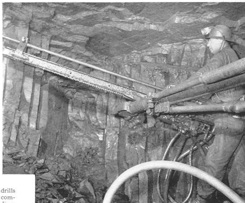
Driller Bill Fitzpatrick operating one of the two drills of a mobile drill unit. Note the advance made by previous drilling round, part of the drill hole still remains. The advance here is 7'4".
